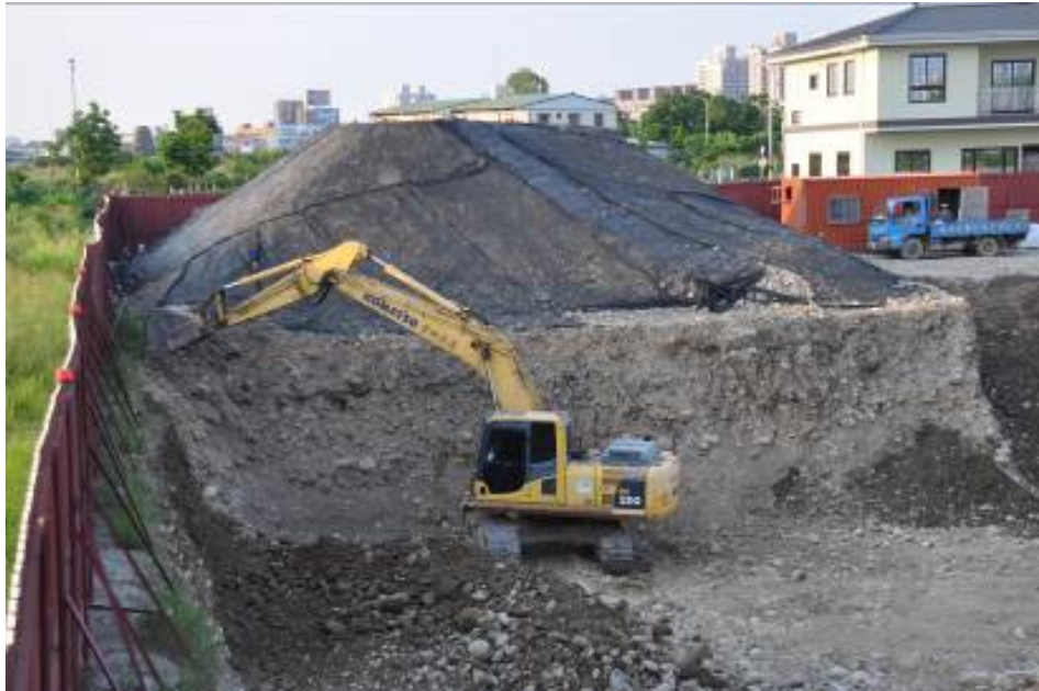
(a) Almost-vertical support-less excavation
